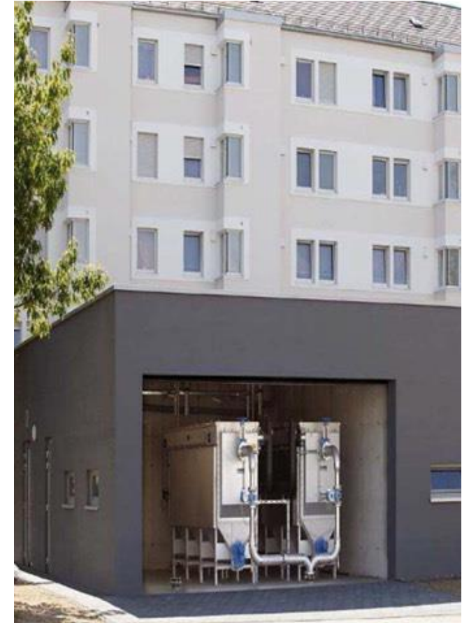
Heat and hot water generated from sewage in Straubing, Germany.
