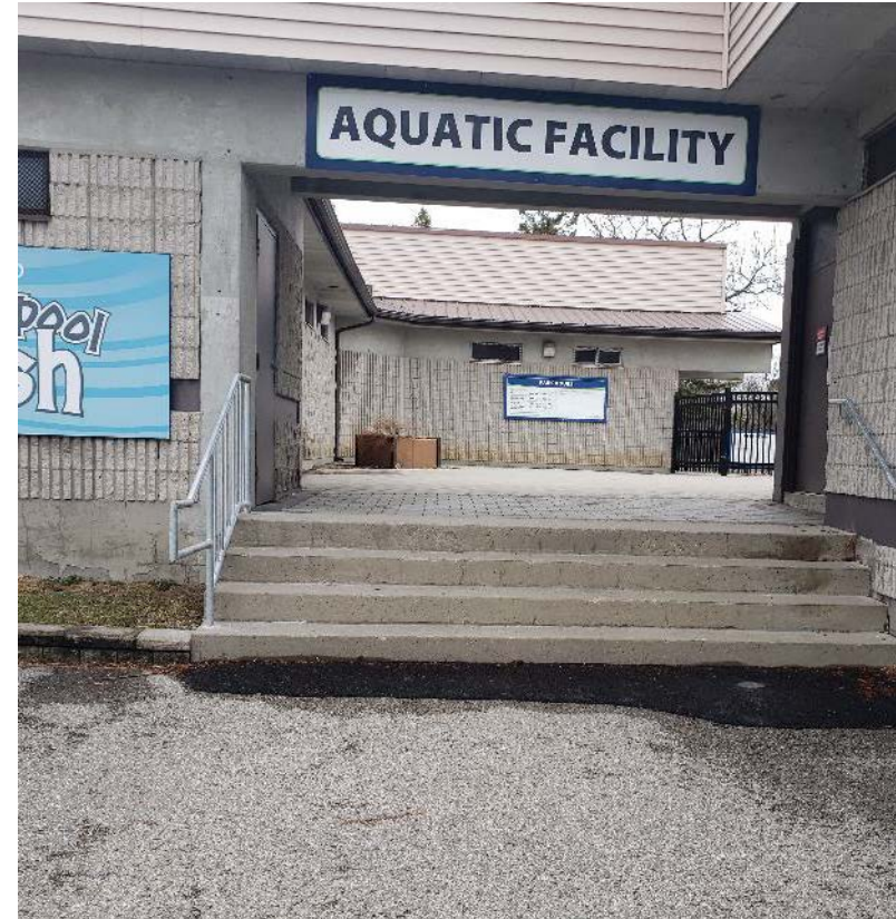
Photo of entrance to the Aquatic Facility. Asphalt settling around concrete stairs. Stairs are steep and narrow. Patch work completed at base of steps and railings installed in attempt to mitigate risk.
