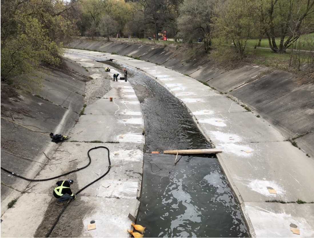
Figure 5 Yonge/York Mills Channel concrete repair in 2020.
