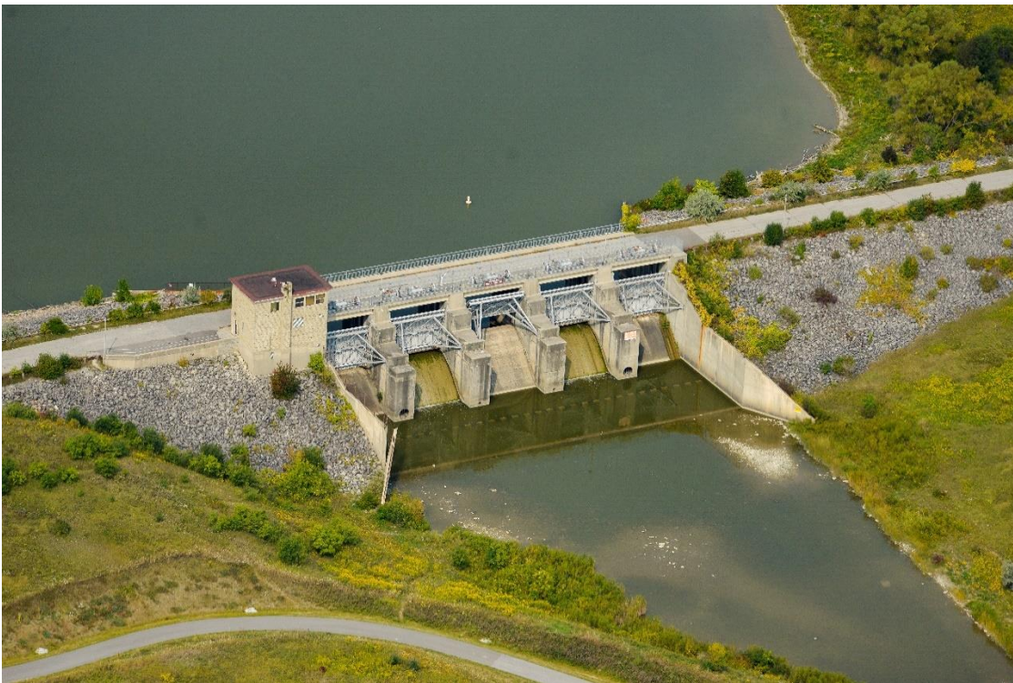
Figure 2 Claireville Dam was constructed in 1963 and requires major maintenance to meet current dam safety guidelines.
