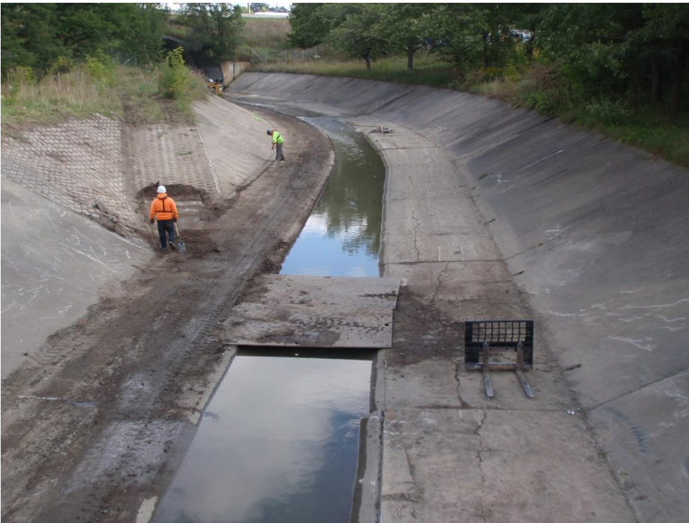
Figure 14 Black Creek Channel after major maintenance (2014).
