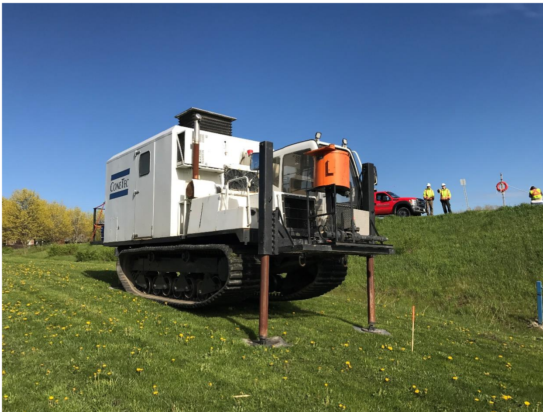
Figure 7 Stouffville Dam undergoing earthquake liquefaction investigation.
