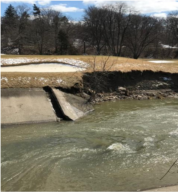
Figure 11 Scarlett Flood Control Channel erosion repair before and after photos.
