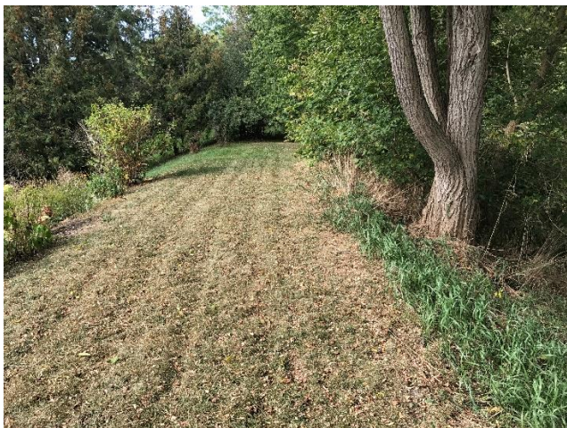
Figure 15 Bolton Berm before major maintenance and upgrades.
