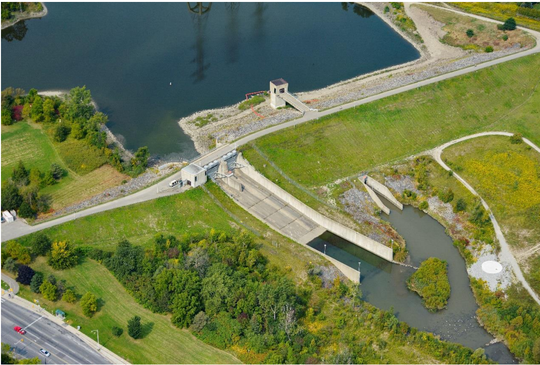
Figure 1 G. Ross Lord Dam carries the highest potential risk of any TRCA dam based on risk to life and property.
