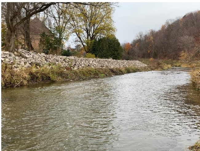
Figure 17 Bolton Berm rip rap installation (2020).
