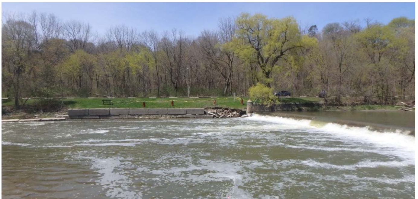
Photograph 1: View of the existing concrete block retaining wall and bank scour along the west bank.
