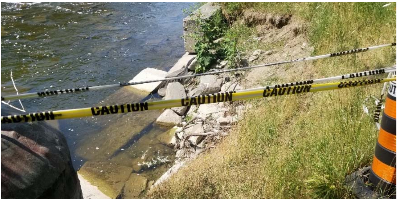
Photograph 2: View of displaced concrete blocks of the retaining wall at the location of the bank scour.
