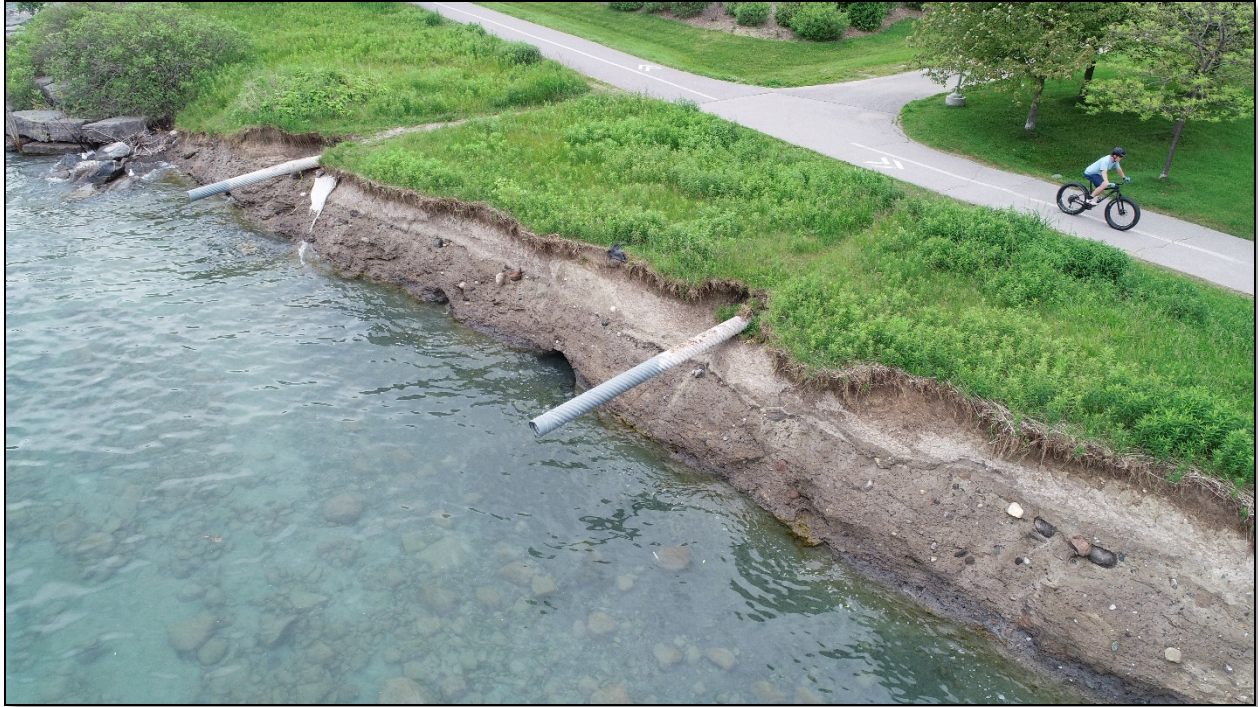
Photo 6: Erosion at Ajax Waterfront Park near Water Supply Plant, Ajax – June 24, 2019
