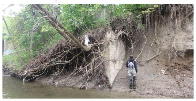
Figure 7. Exposed manhole chamber along Black Creek, City of Toronto.
