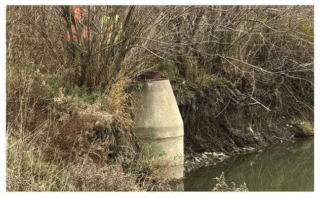
Figure 4. Exposed manhole chamber along Rainbow Creek Site 2.
