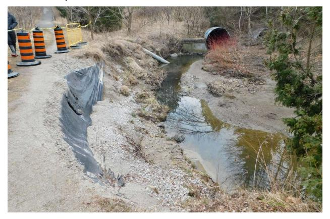
Figure 8. Eroding bank and trail along Newtonbrook Creek, City of Toronto.
