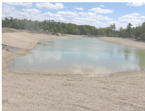
Figure 7.8: Temporary sediment control pond
