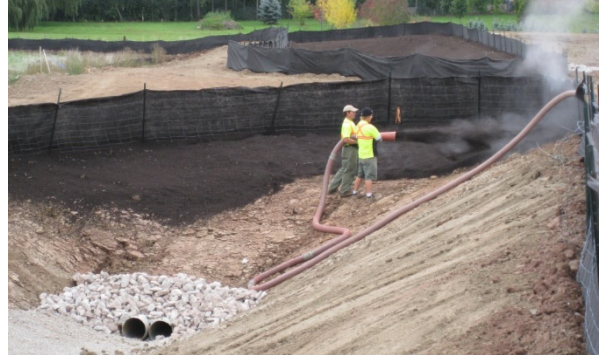
Figure B1-11: Pneumatic seeding with growing media
