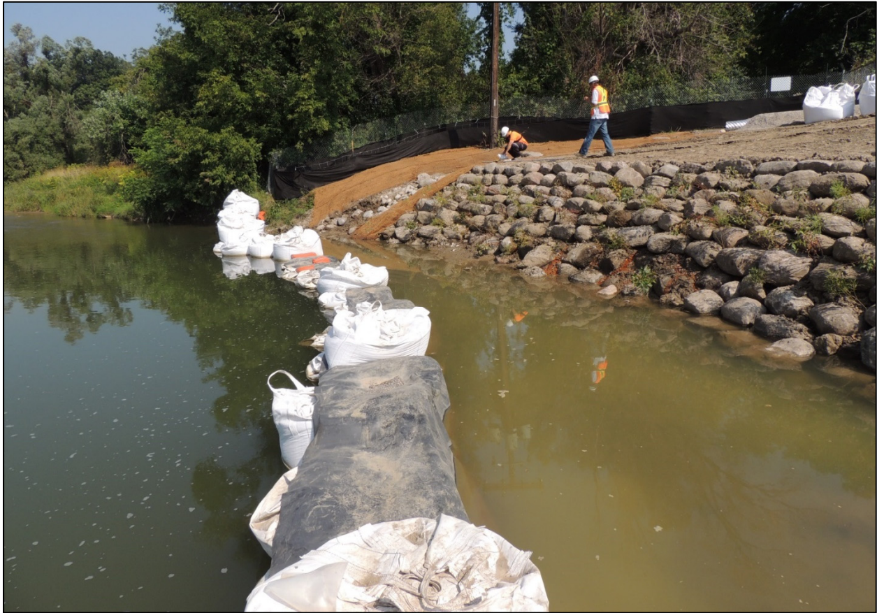
Figure C5: Waterproof isolation barrier (cofferdam)
