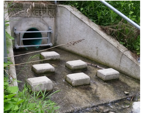
Figure B1-12: Erosion blanket in an outlet area (top) and baffle blocks for energy dissipation (bottom)
