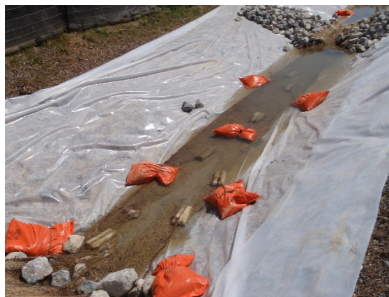
Figure 7.11: Polymer-based treatment train in a dewatering ditch
