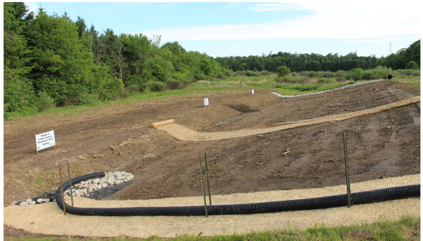
Figure B1-3: Slope drain
