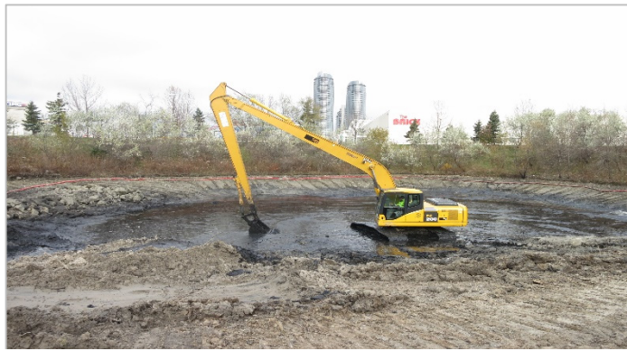
Figure B2-20: Sediment removal from a pond
