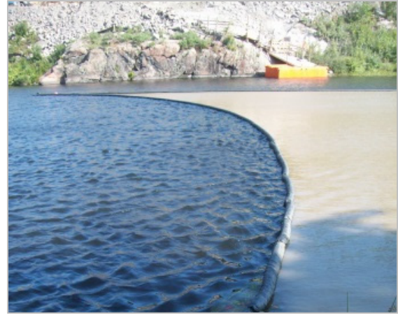
Figure 7.15: Turbidity curtain applied to isolate a work area when working in the wet
