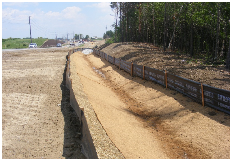
Figure B1-4: Stabilized interceptor swale
