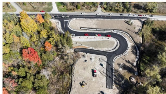
Construction of the new entrance to Bolton Camp
