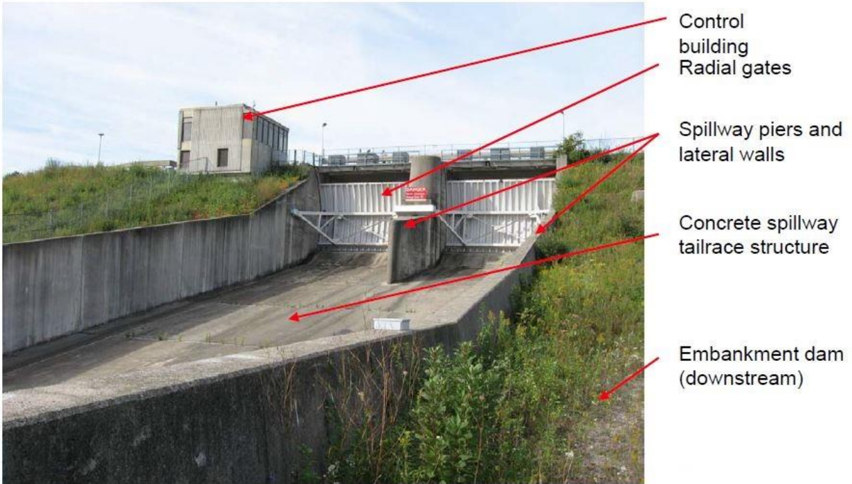
Figure 8.2 - G. Ross Lord Dam Emergency Spillway
