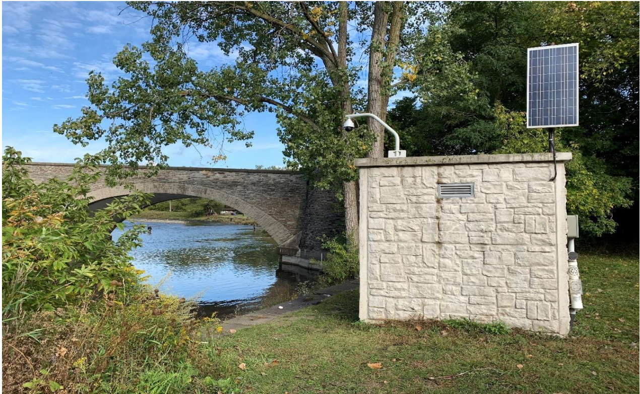
Figure 8.4 - Old Mill at Humber River Real-time Stream Gauge
