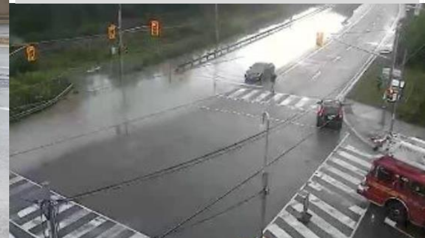
Flooding on Bayview Ave. extension near Pottery Rd, Toronto – August 17
