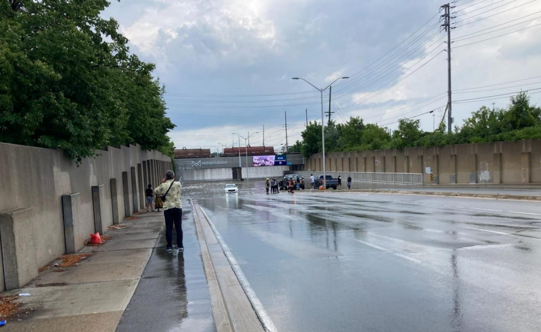
Railway bridge overpass, Dixie Rd south of Dundas St., Mississauga – August 17. Photo credit: G. MacDonald
