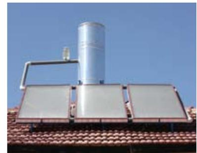
water-heating systems directly substitute renewable energy for conventional energy, reducing the use of electricity or natural gas by as much as 80 per cent.
