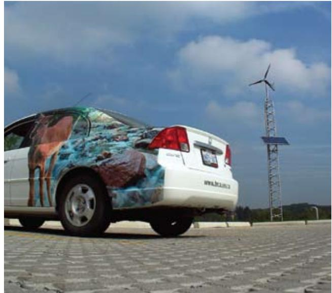
Permeable pavement is a way to treat stormwater onsite and improve local water quality.
