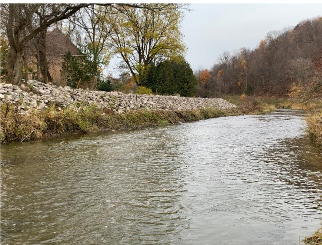
**Figure 17** Bolton Berm rip rap installation (2020).
