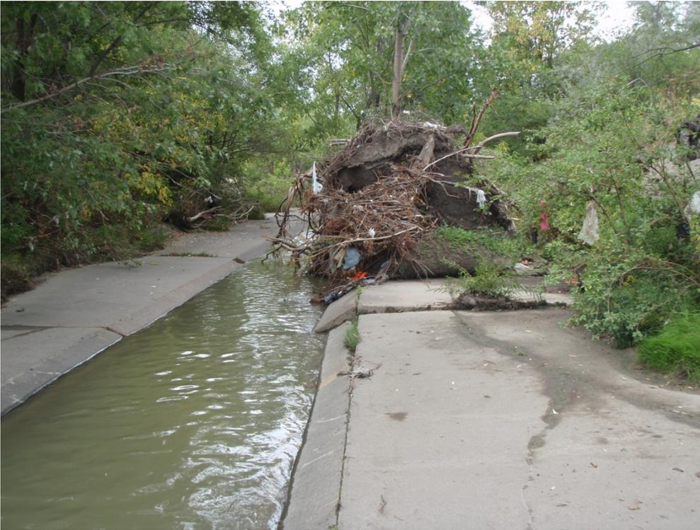
**Figure 13** Partially blocked flood control channel at Black Creek.
