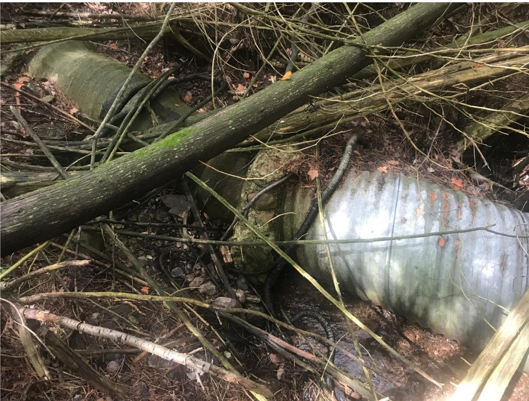
**Figure 4** Failed spillway pipe at Glen Haffy Fly Fishing Upper Dam
