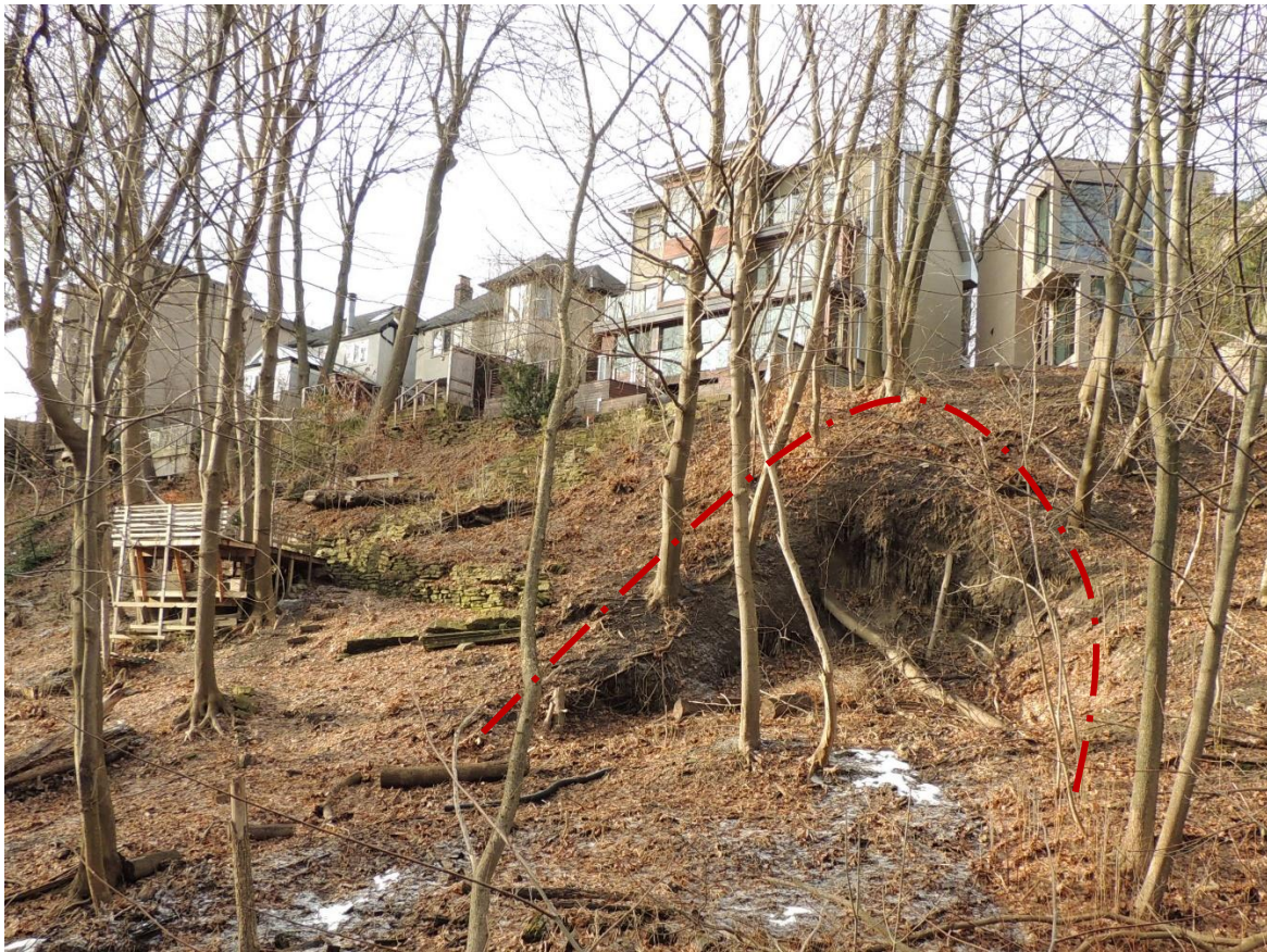
Figure 1. View of the slope failure from the Beltline Trail facing southwest towards 193 – 195 Hudson Drive. Red dashed line highlighting slope failure. Source: TRCA 2018
