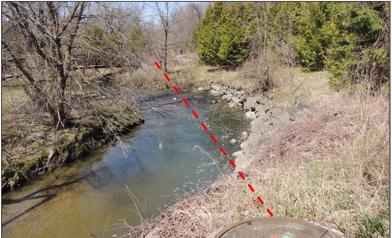
Figure 2. The Leslie Collector main and maintenance hole is at risk of erosion downstream of the pedestrian bridge in German Mills Settlers Park. Source: TRCA, 2018.
