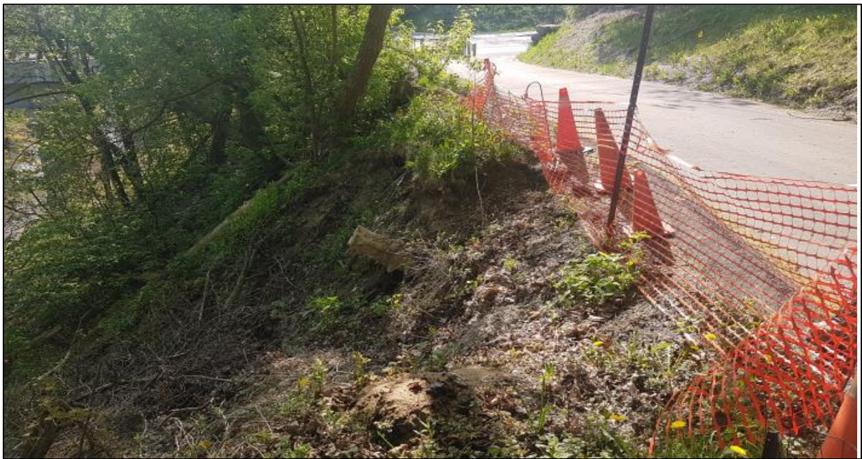
Figure 2. Slope crest with view of bare and unvegetated erosion scour on the slope crest facing east towards the Main Street South roadway.
