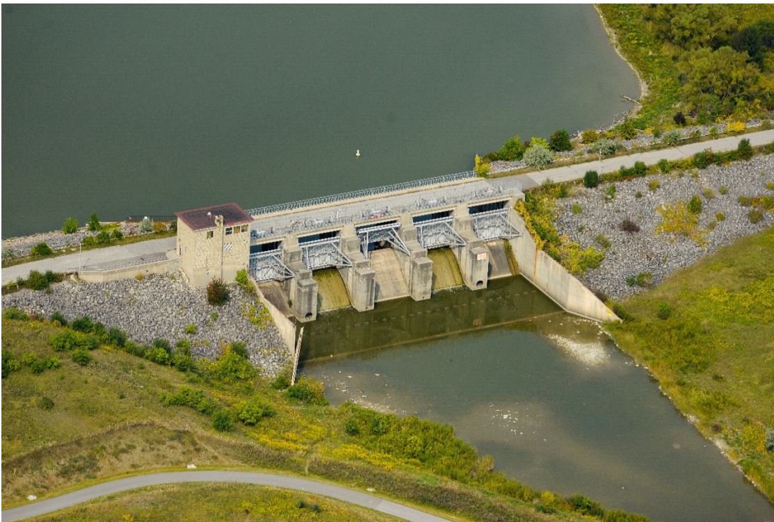
Figure 2 Claireville Dam looking upstream.
