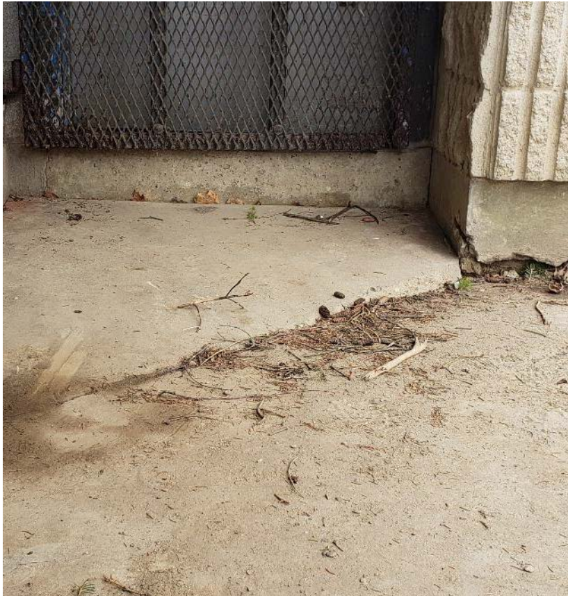
Photo of the entrance to washroom building. Eroding building structure. Heaved and broken concrete creating accessibility issues so that wheelchairs cannot enter.
