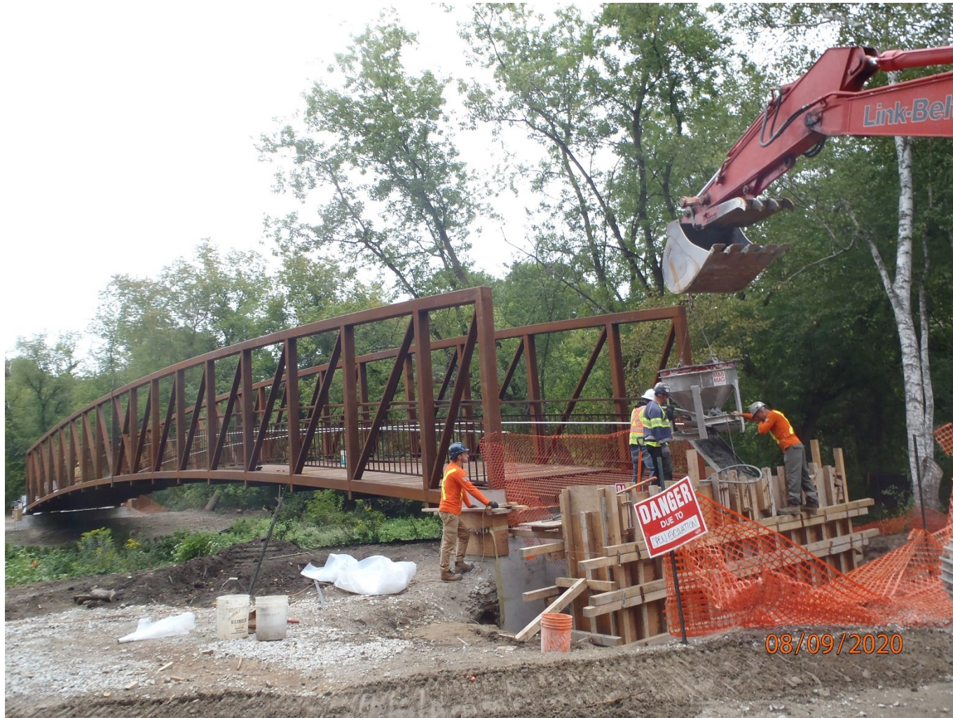
Bridge 2 south ramp abutments footing works (west of the rail line and future tunnel)
