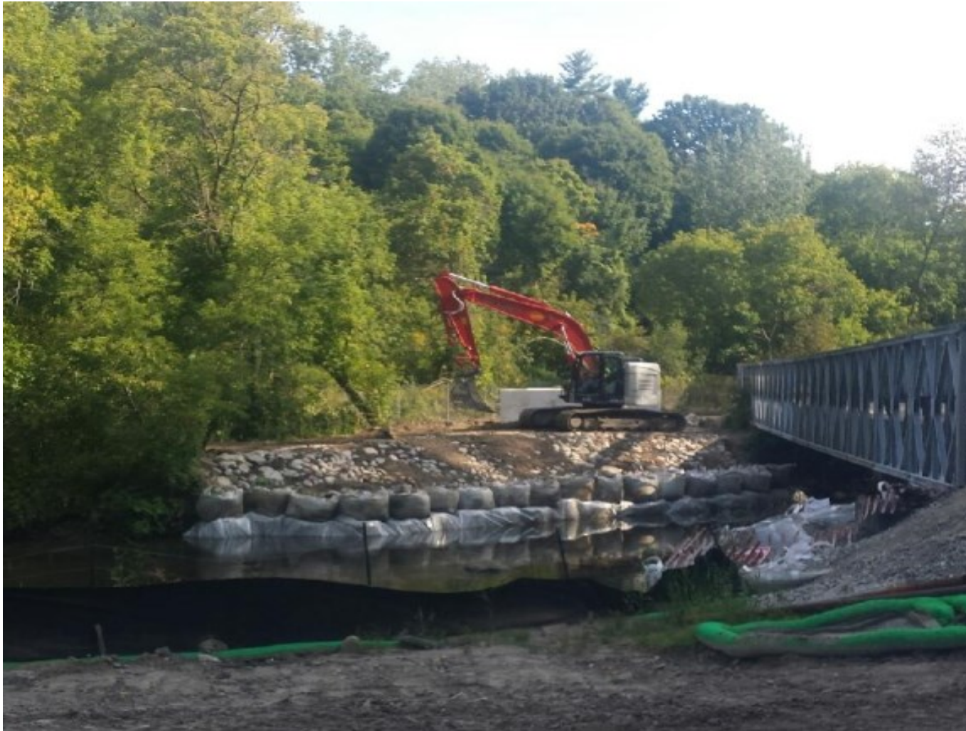
Bank stabilization at bridge crossing over the East Don River completed in Fall 2019
