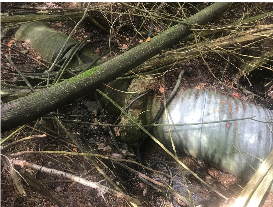
Figure 4 Failed spillway pipe at Glen Haffy Fly Fishing Upper Dam
