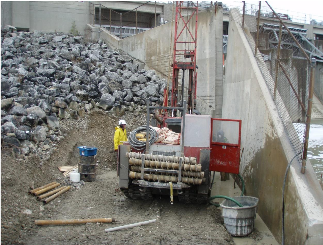
Figure 3 Claireville Dam wing wall settlement investigation.
