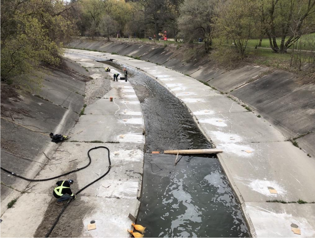
Figure 5 Yonge/York Mills Channel concrete repair in 2020.
