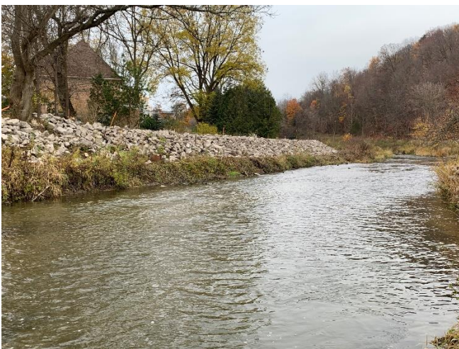
Figure 17 Bolton Berm rip rap installation (2020).
