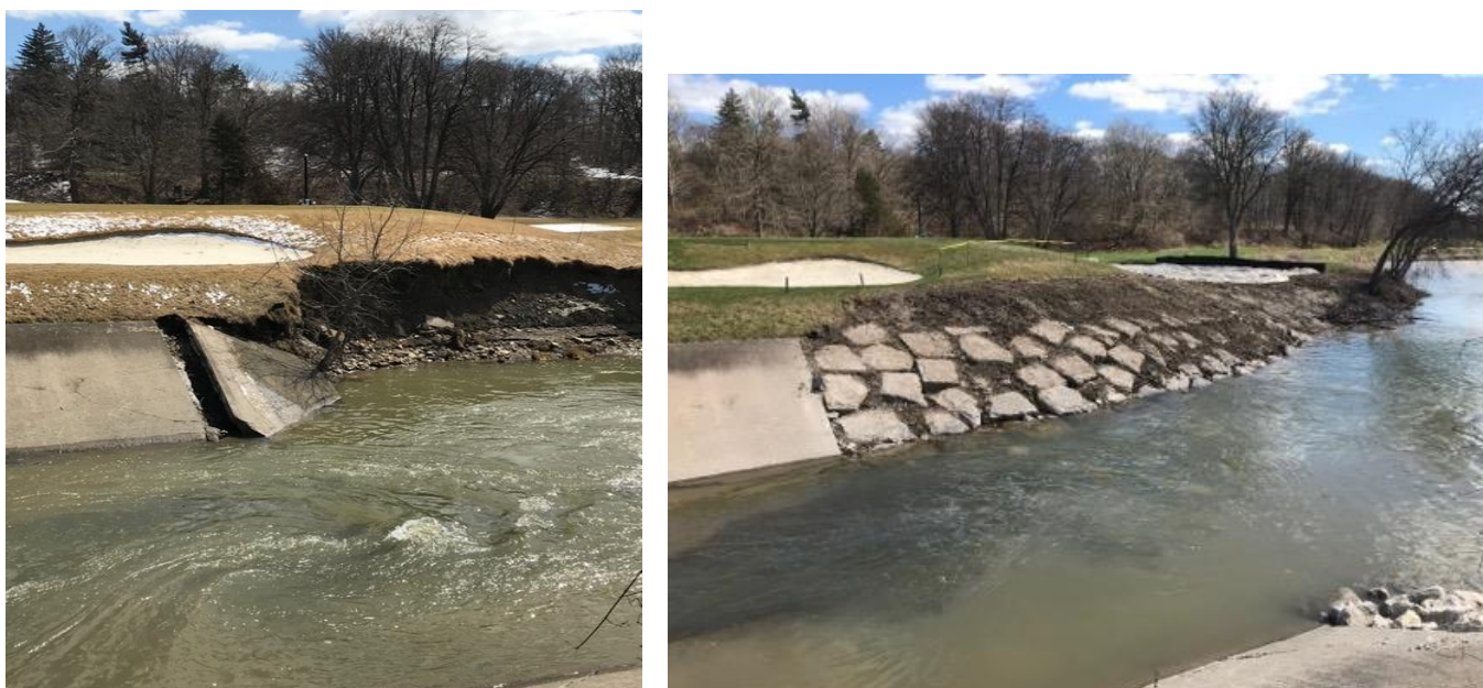
Figure 11 Scarlett Flood Control Channel erosion repair before and after photos.
