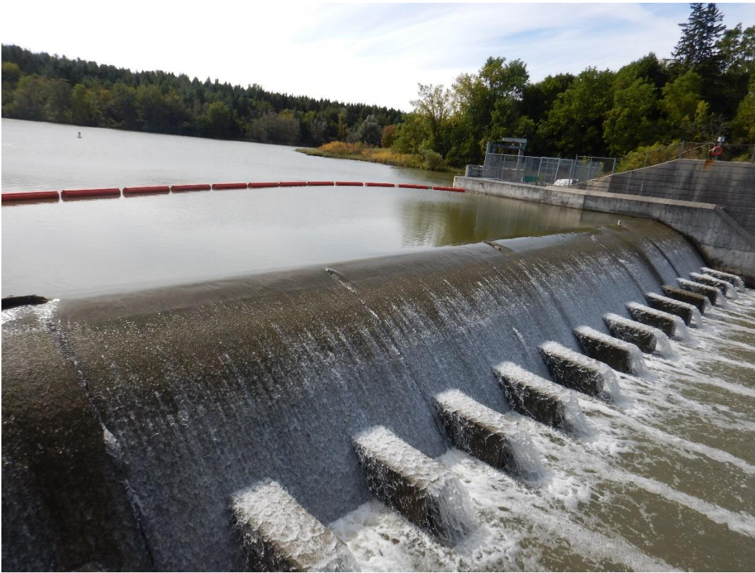
Figure 9 Milne Dam's spillway is too small for extreme floods and requires upgrades to withstand overtopping.
