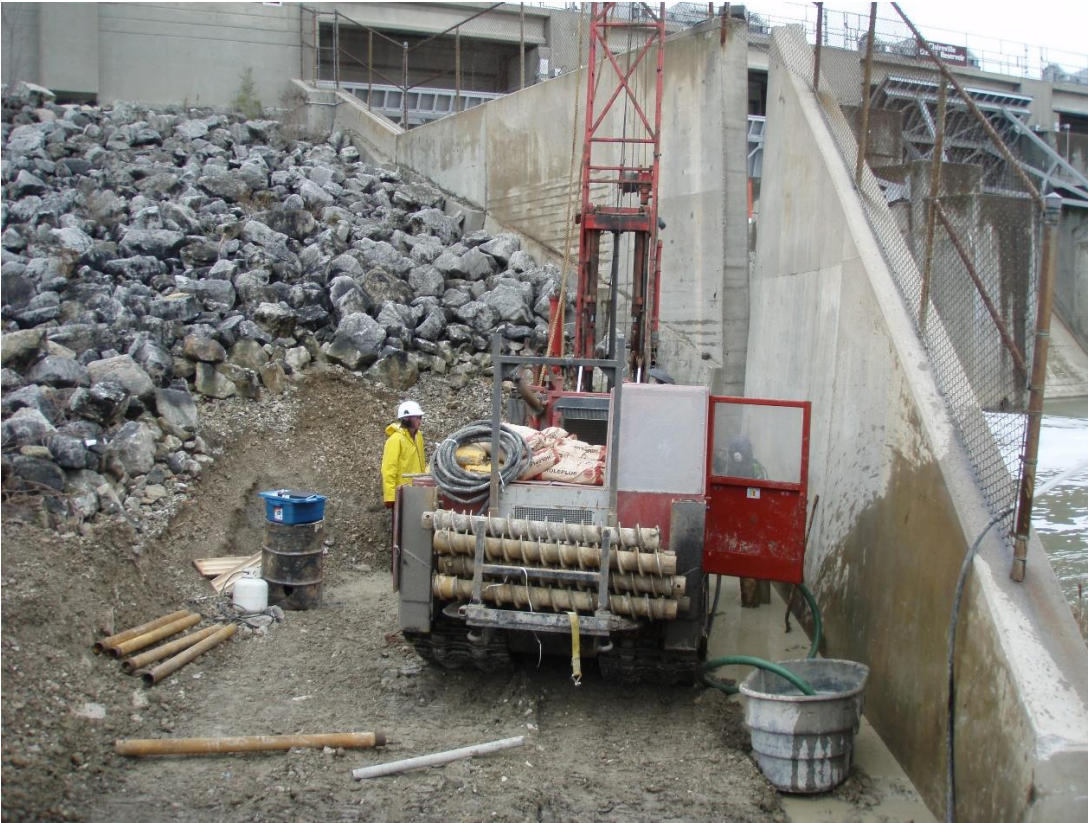
Figure 3 Claireville Dam wing wall settlement investigation.
