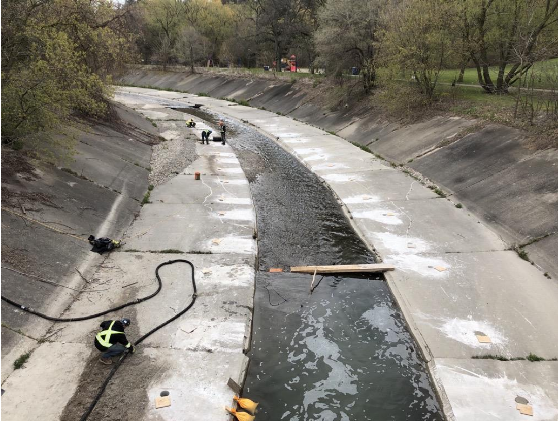
Figure 5 Yonge/York Mills Channel concrete repair in 2020.
