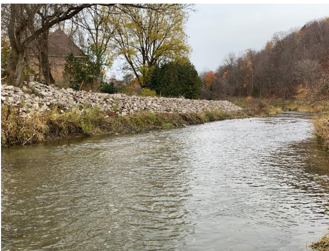
Figure 17 Bolton Berm rip rap installation (2020).
