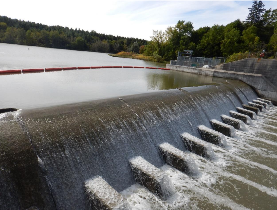
Figure 9 Milne Dam's spillway is too small for extreme floods and requires upgrades to withstand overtopping.
