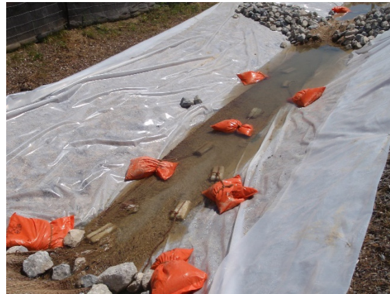
Figure 7.11: Polymer-based treatment train in a dewatering ditch
