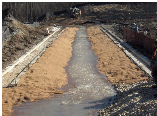
Figure 9.1: Watercourse diversion during construction is exempt from requiring a PTTW.
