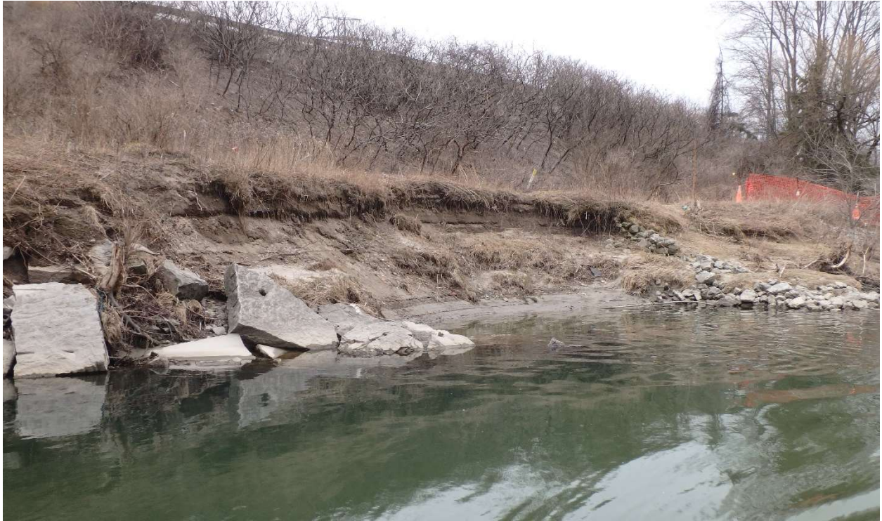
Figure 1. Eroding bank at failed TRCA erosion control asset along the main branch of the Don River, City of Toronto.
