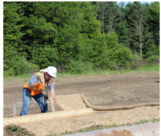
Figure B1-15: RECP installed on a slope and anchored in place at the top
