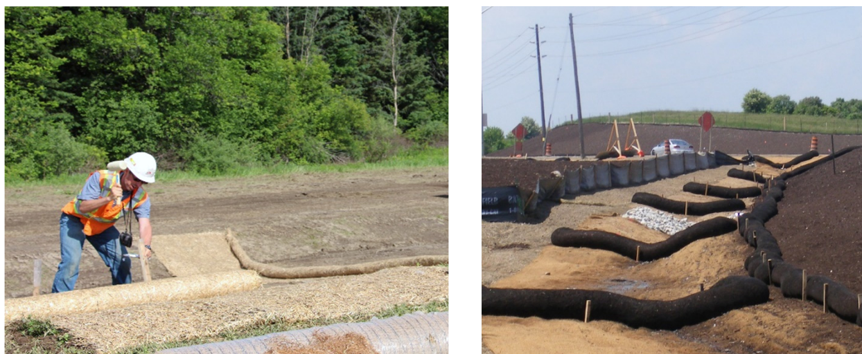
Figure 4.6: Erosion control blanket (left) and filter socks applied as sediment control check dams (right).
