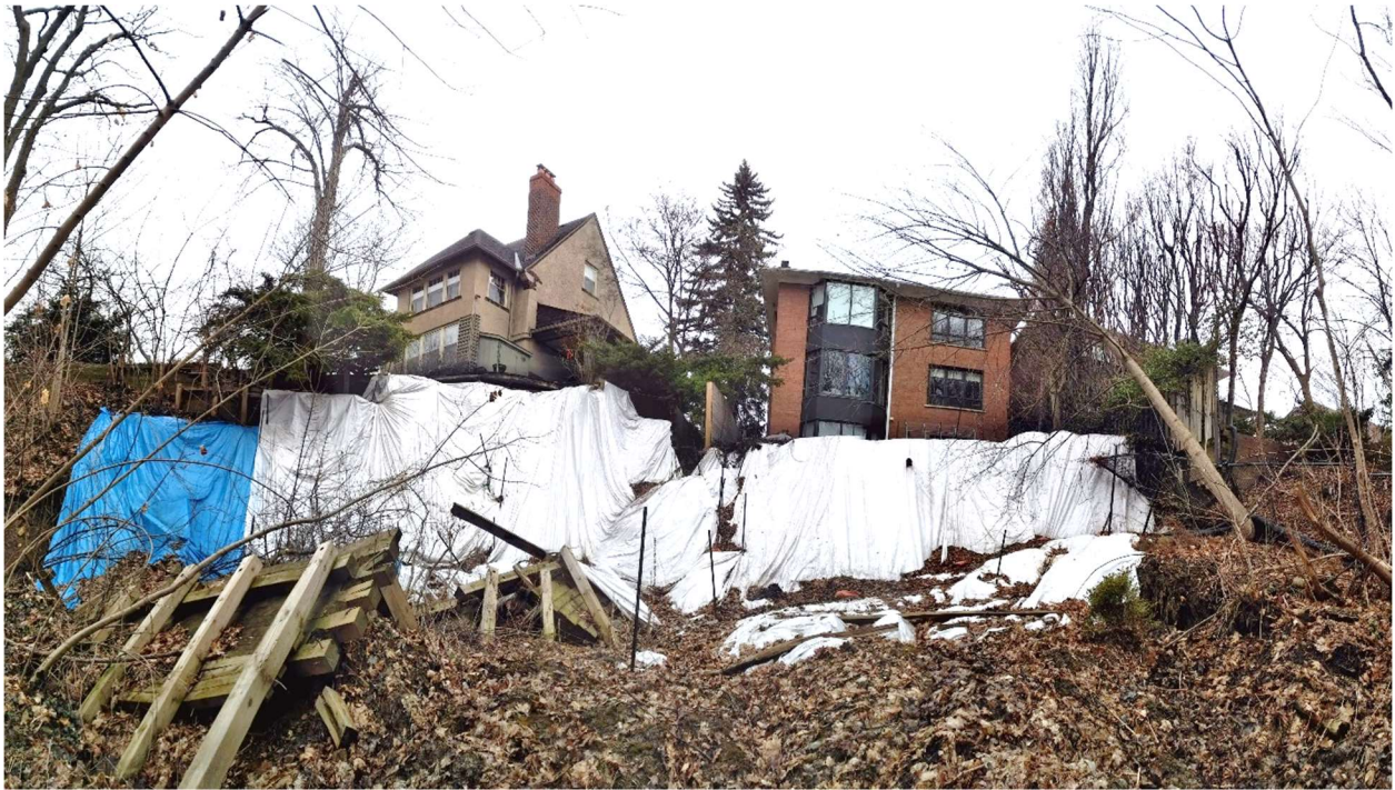
Figure 3. Slope failure at a Valley Erosion Hazard Site in the City of Toronto.
