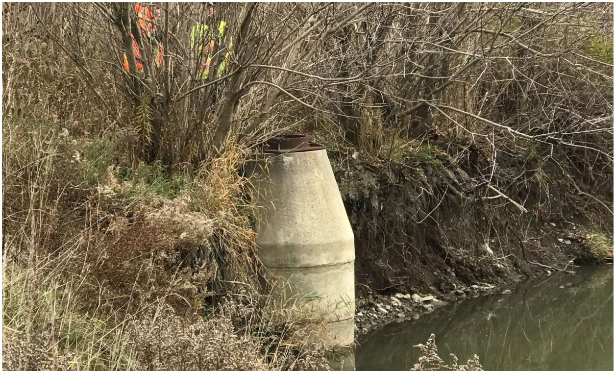
Figure 4. Exposed manhole chamber along Rainbow Creek Site 2.
