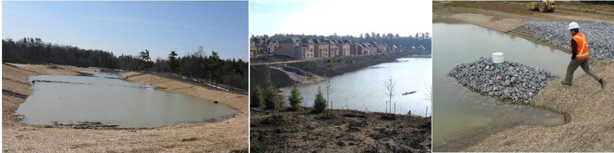
Figure B2-19: Sediment control ponds
