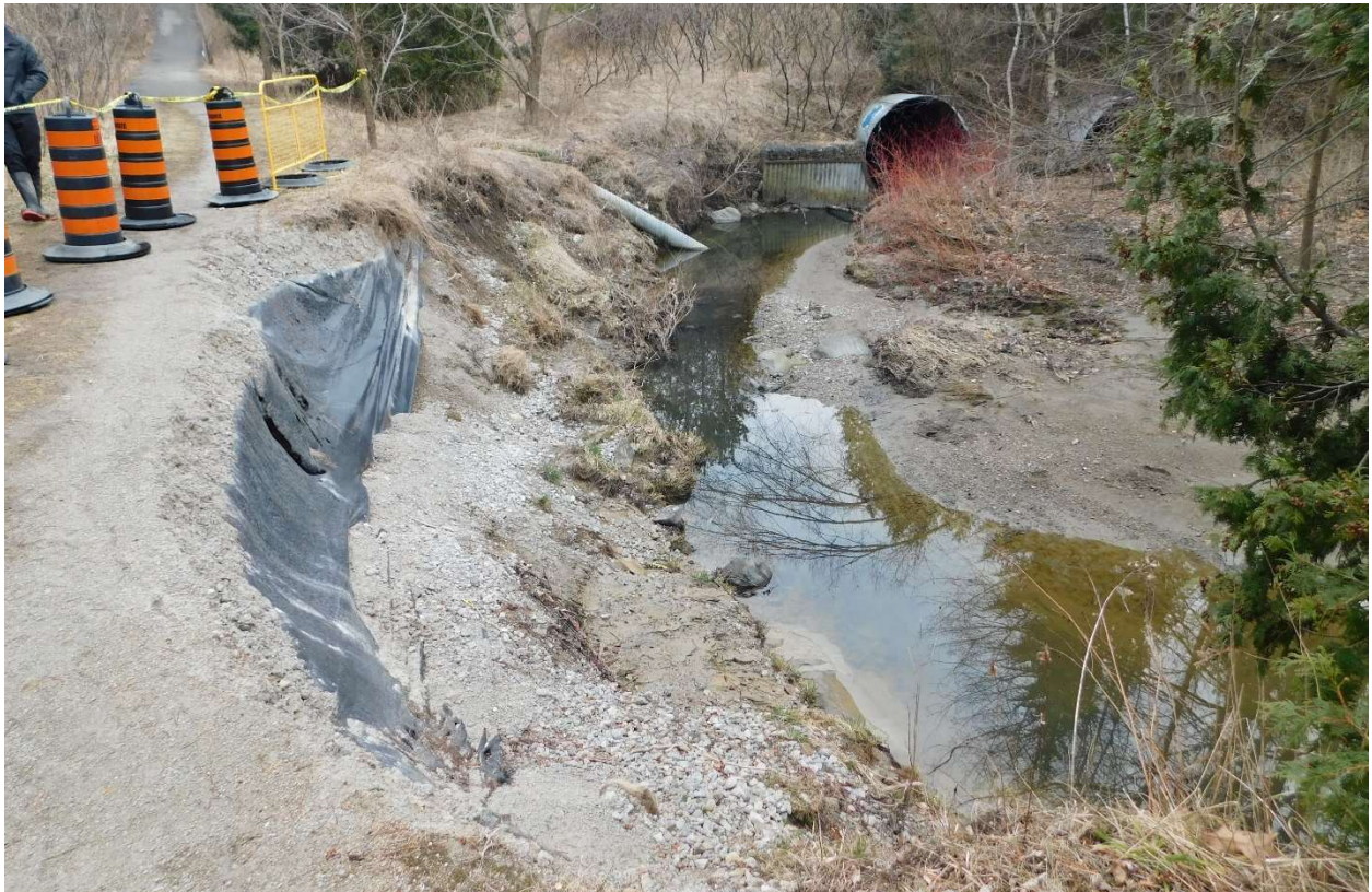
Figure 8. Eroding bank and trail along Newtonbrook Creek, City of Toronto.
