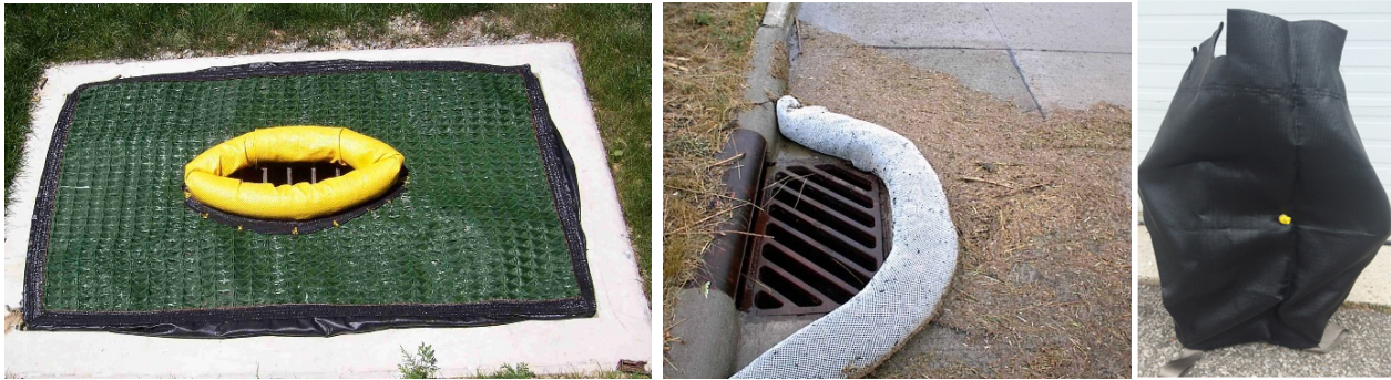
Figure B2-12: Storm drain inlet protection measures
