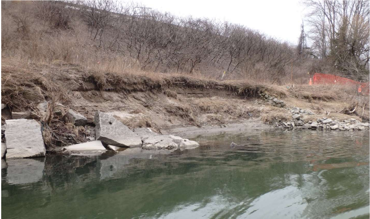
Figure 1. Eroding bank at failed TRCA erosion control asset along the main branch of the Don River, City of Toronto.
