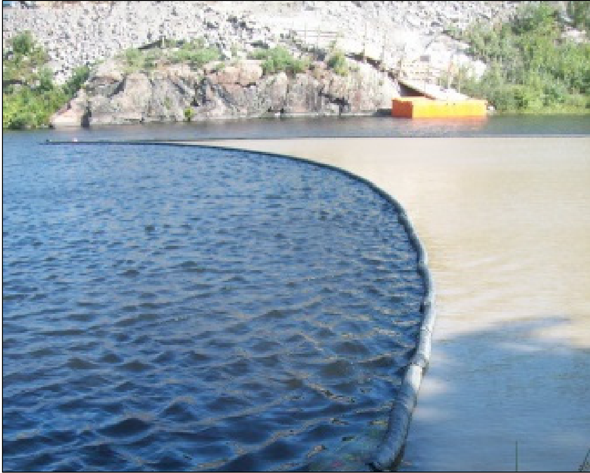
Figure C2: Sediment curtain installed in a lake
