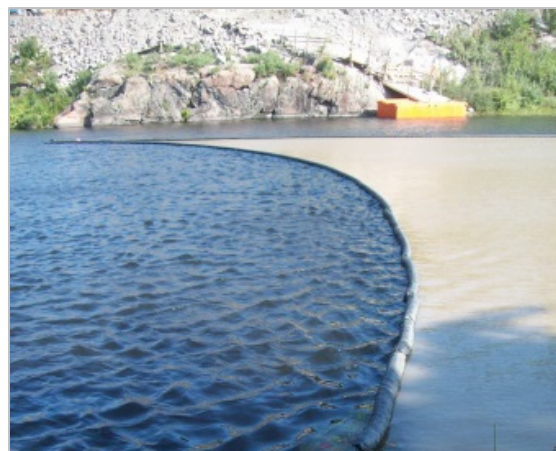
Figure 7.15: Turbidity curtain applied to isolate a work area when working in the wet
