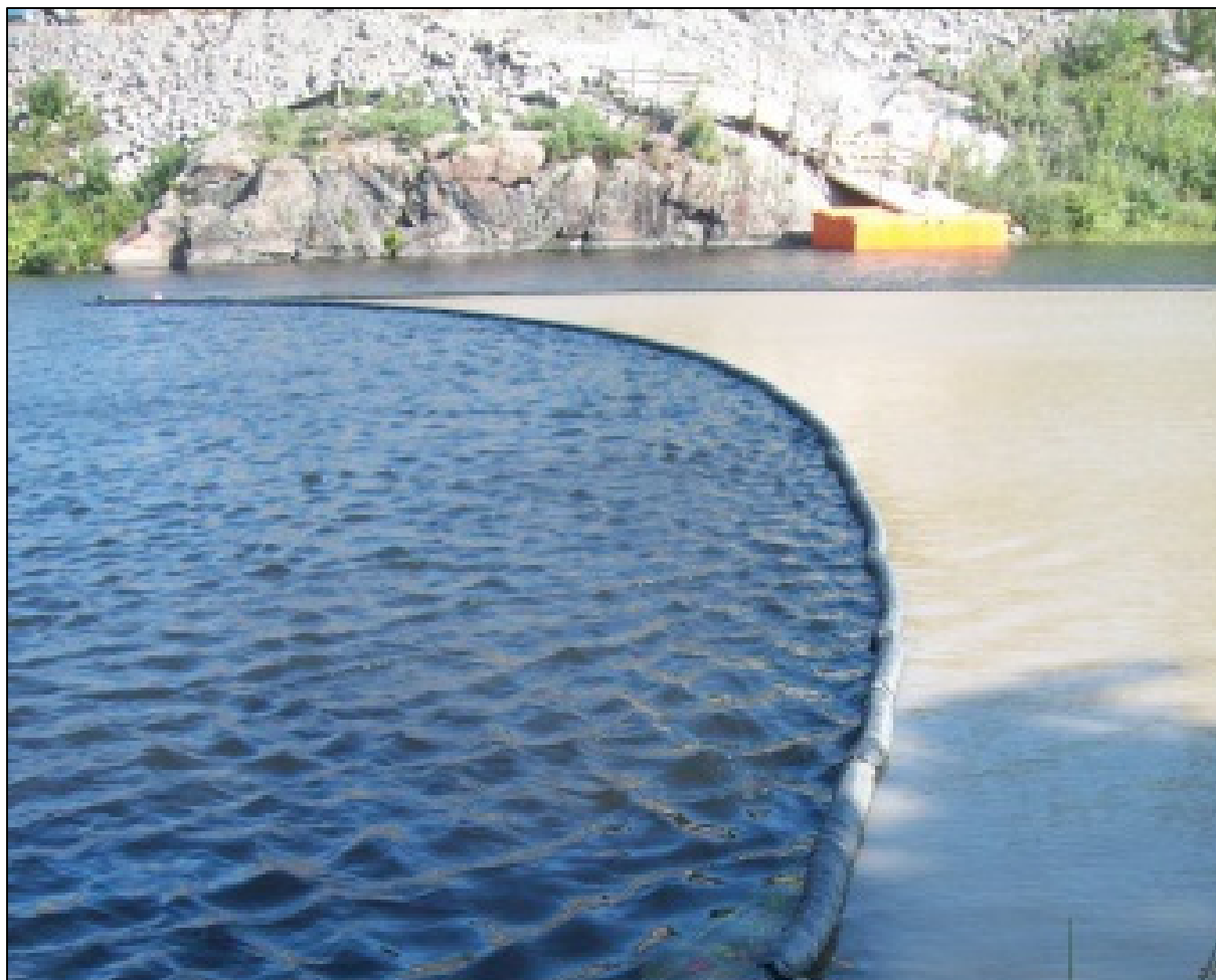
Figure C2: Sediment curtain installed in a lake
