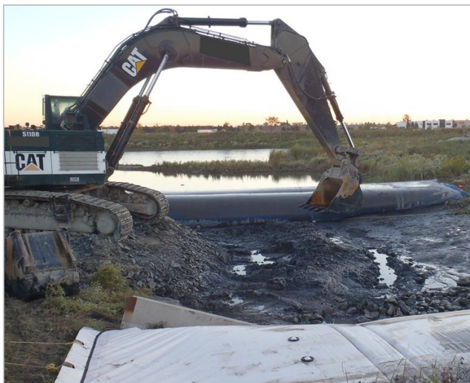
Figure 7.14: In-water worksite isolation
