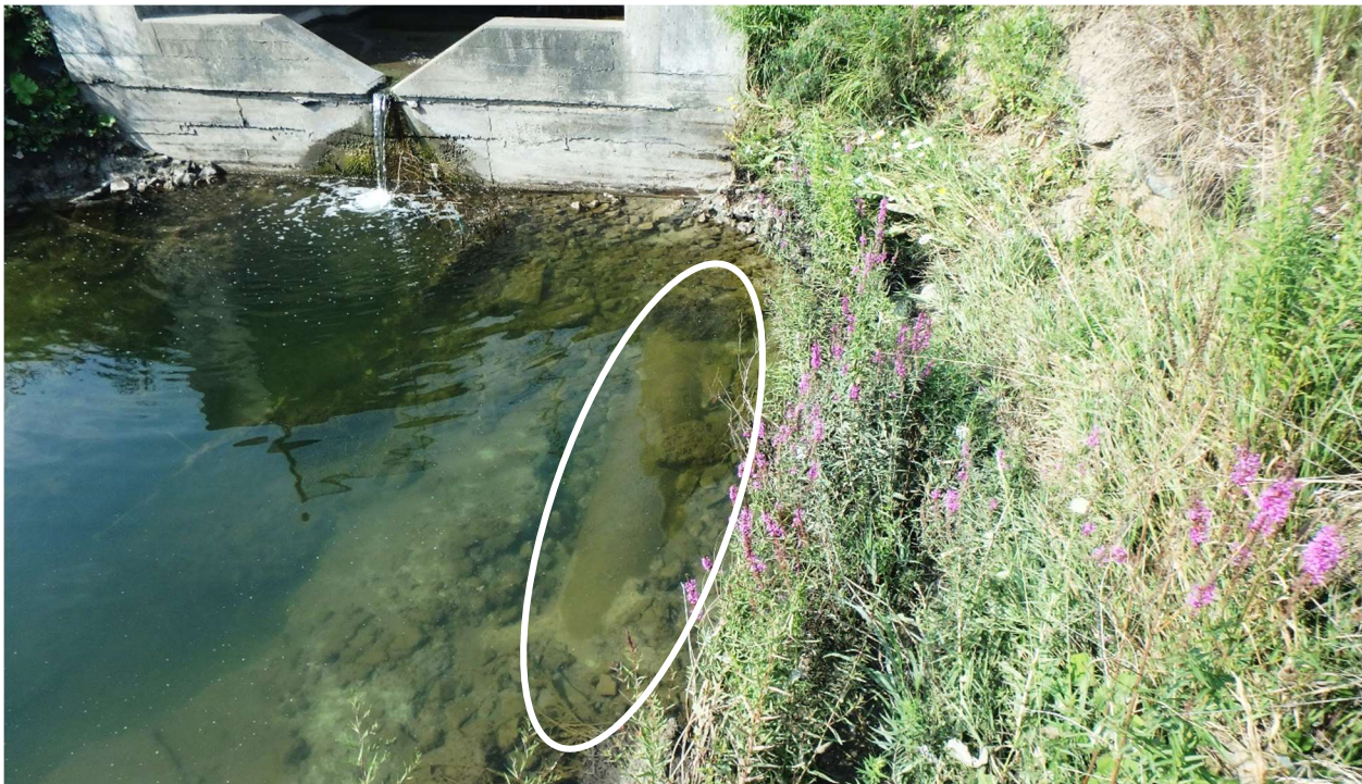
Figure 6. Exposed sanitary sewer (circled) at Region of Peel Infrastructure Site P-315.
