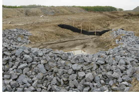
Figure B2-9: Rock check dam
