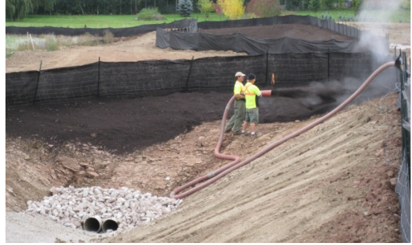
Figure B1-11: Pneumatic seeding with growing media
