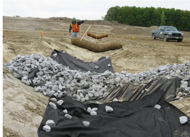
Figure 10.7: Maintenance of rock check dams
