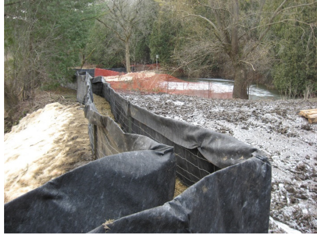
Figure B2-2: Double row sediment control fencing
