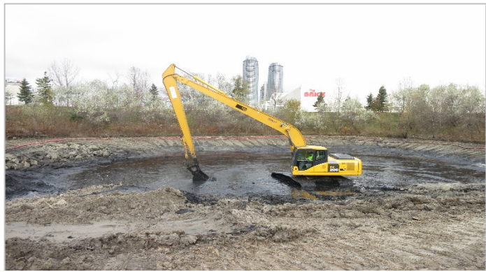
Figure B2-20: Sediment removal from a pond
