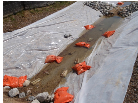
Figure 7.11: Polymer-based treatment train in a dewatering ditch
