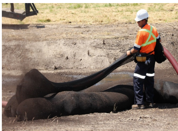
Figure B2-4: Filter sock being filled on site
