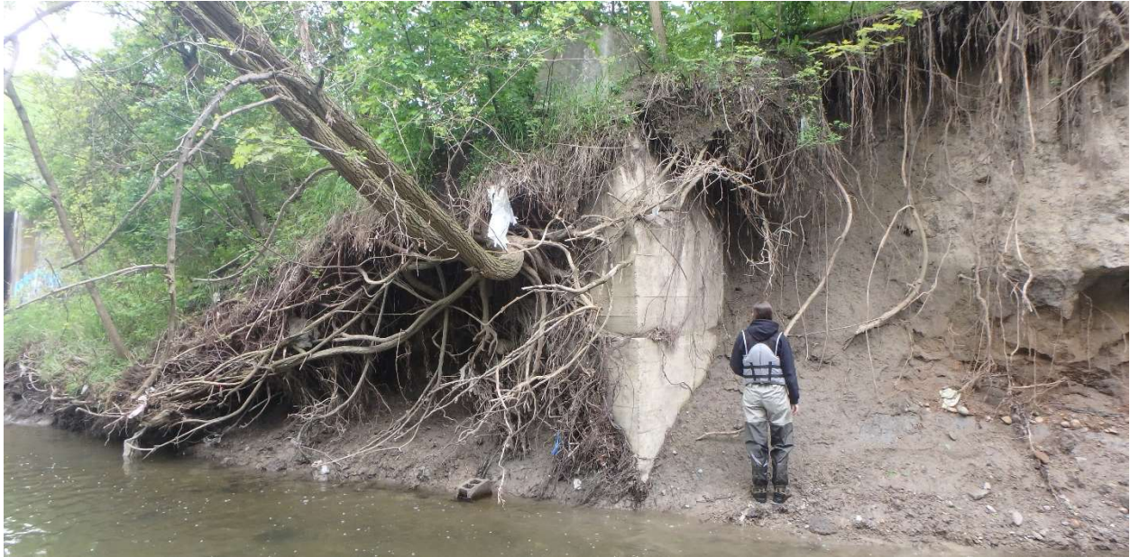
Figure 7. Exposed manhole chamber along Black Creek, City of Toronto.
