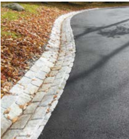
Permeable swales at roadways
