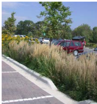
Curb with openings to allow drainage to bioswales, Durham College, UOIT
