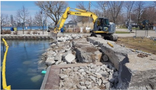
Emergency works at Toronto Island in response to 2019 flooding.
