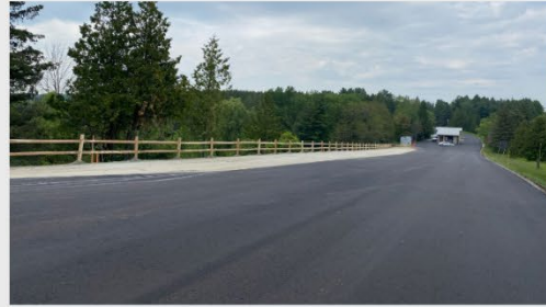
Newly paved roadway at Albion Hills Conservation Park
