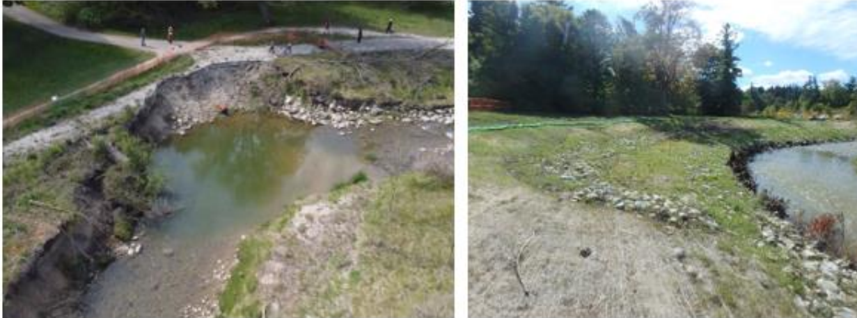
Figure 7.4 - Former erosion hazard at Boyd Conservation Area captured by mRPAS before construction of a new erosion control system (before on the left photo, and after on the right photo). Source: TRCA, 2021.
