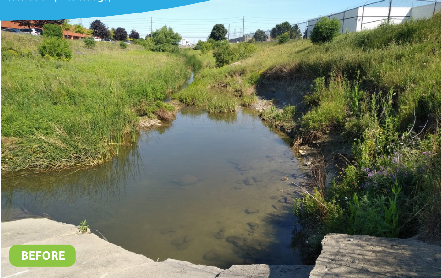
FIGURE 8: Before and After, Kings Park Stream Restoration (Mississauga)
