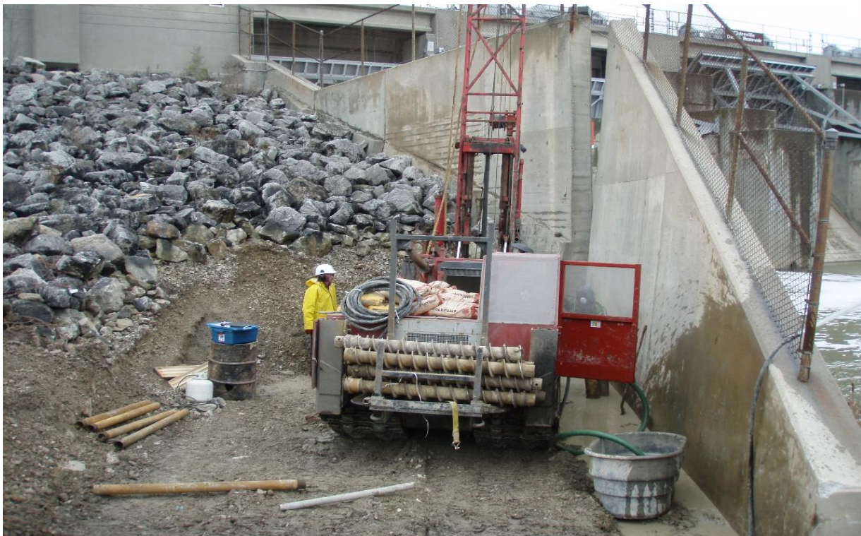
Figure 8.11 - Geotechnical drilling at Claireville Dam's downstream wing wall
