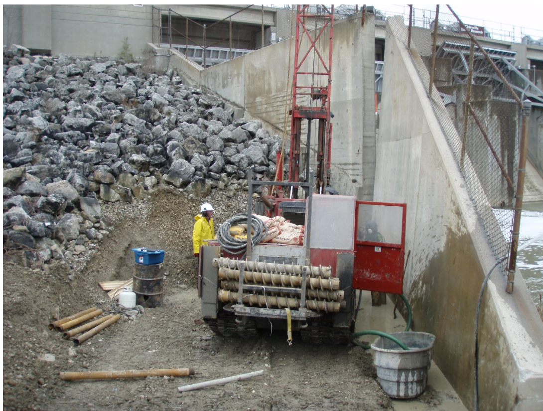
Figure 3 Claireville Dam wing wall settlement investigation.
