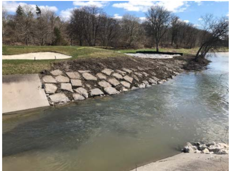
Figure 11 Scarlett Flood Control Channel erosion repair before and after photos.
