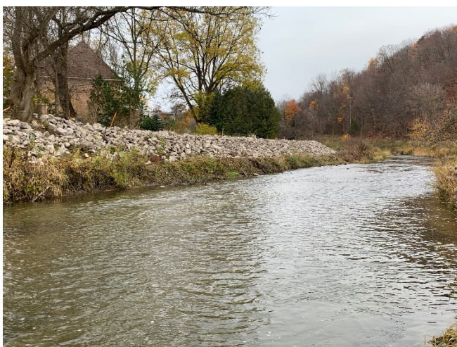
Figure 17 Boltan Berm rip rap installation (2020).
