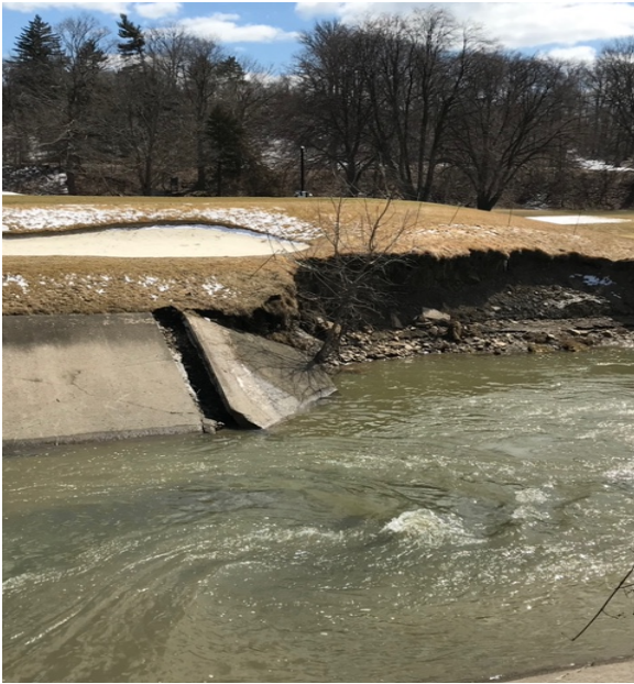
Figure 11 Scarlett Flood Control Channel erosion repair before and after photos.
