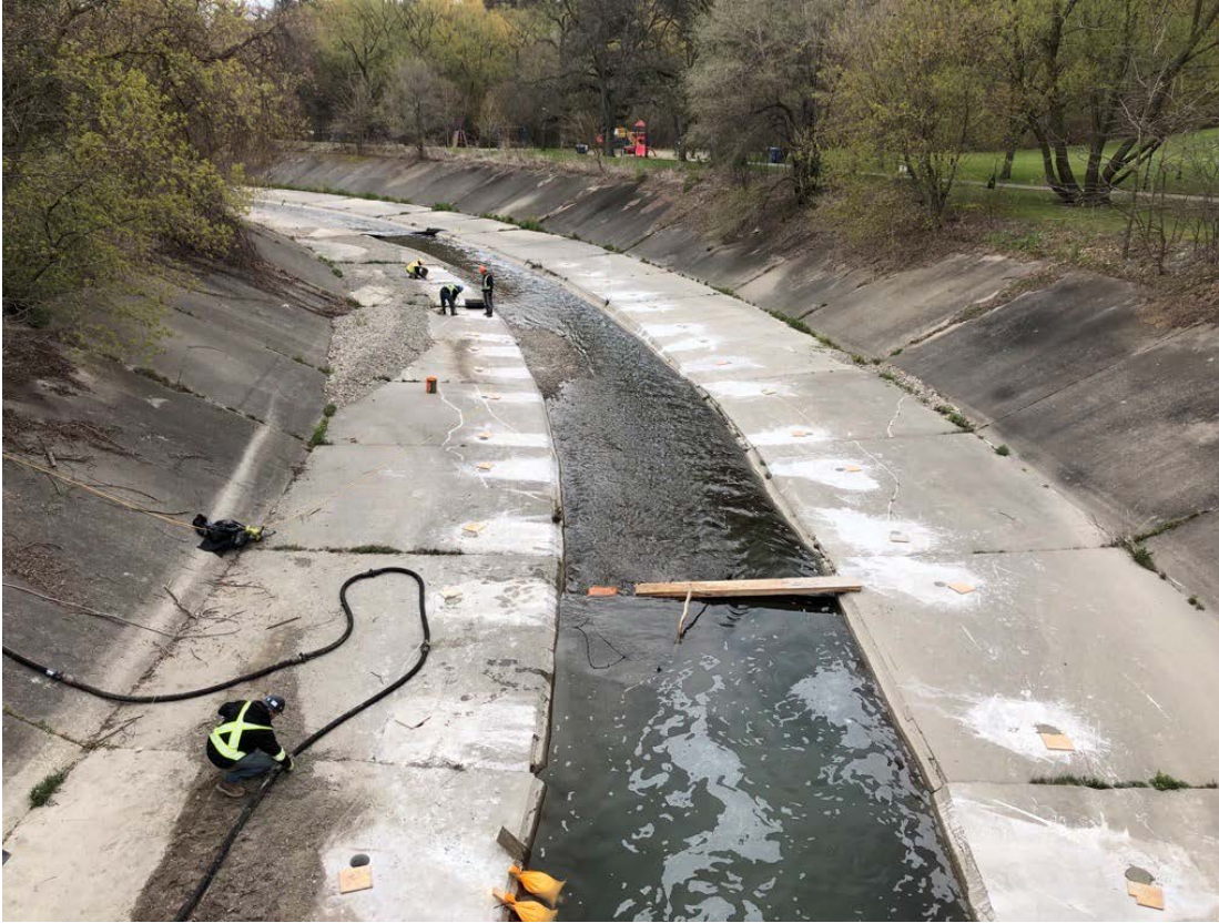
Figure 5 Yonge/York Mills Channel concrete repair in 2020.
